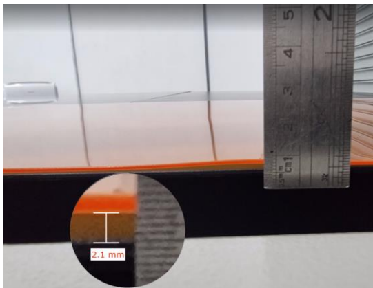
Figure 3 High wave that exceeds the acceptable tolerance (the measured wave is > 1.5 mm).
